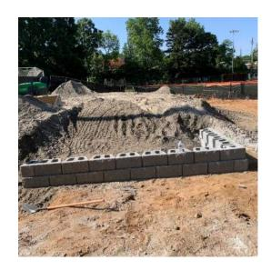
East Elevation Retaining Wall
